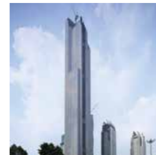
POWER SYSTEMS Guangzhou CTF Finance Center & Rosewood Hotel Page 59
