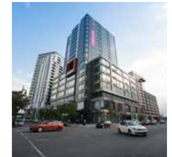
CONSTRUCTION MANAGEMENT District Griffintown – Block 10 Page 49
