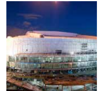
GEOTECHNICAL ENGINEERING Tele2 Arena Page 42
