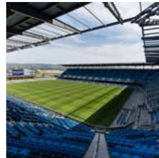
COMMISSIONING Avaya Stadium Page 39
