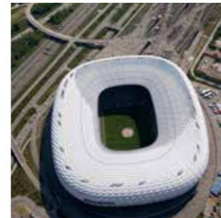
CONSTRUCTION MANAGEMENT Allianz Arena Page 15
